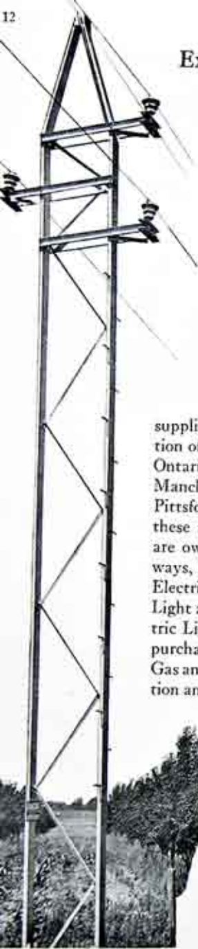
Steel Towers on the Canandaigua Transmission Line
