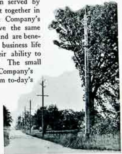
Wooden Poles as used on a Narrow Right-of-Way in Canandaigua.
