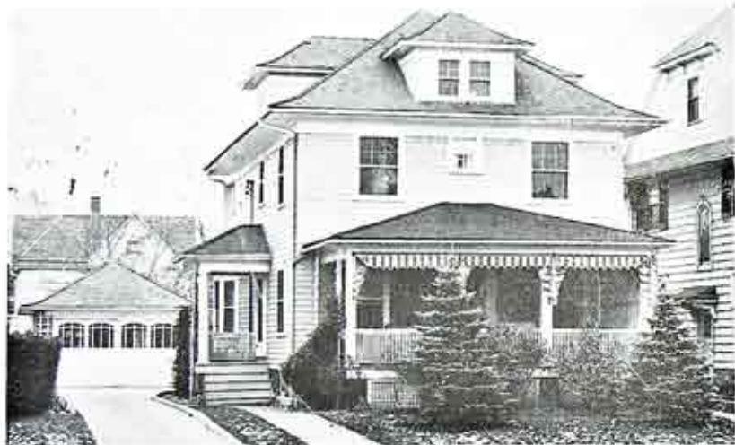
Fig. 6: Mr. J. J. Ottman's Residence, 44 Crosman Terrace, Which Is Being Heated by the Hot Water Boiler Shown in Fig. 4.
