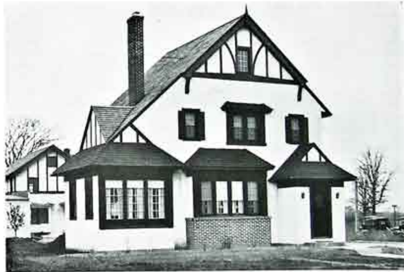
Fig. 7: Home of Mr. I. E. La Grange, 28 Navarre Road, in Which the Hot Air Gas Furnace Shown in Fig. 2 Is Now in Operation.
