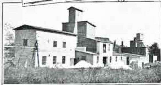
5—Bo Brick Kept These Walls Up. 6—Steel Failed But Bo Brick Endured Intense Heat 7—Clay Brick Chimney Collapsed. 8—The Harrisburg, Pa., Plant.
