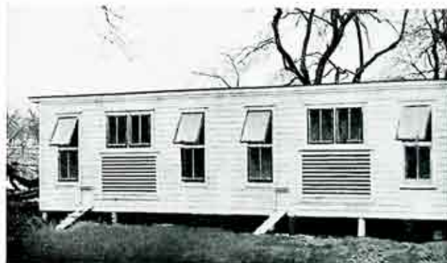
Fig. 3.—A Modern Electrically Lighted Poultry House
