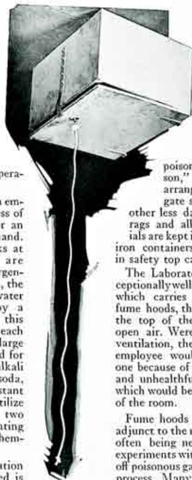
Fig. 2: Merely Pull the Cord and a Blanket is Released from the Box on the Ceiling
