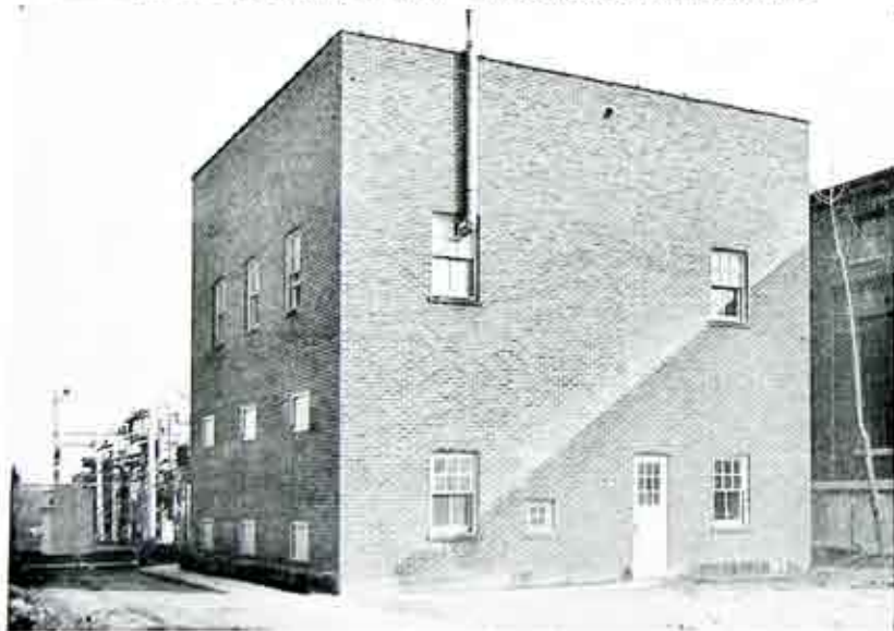
Fig. 5: Station 36, Charlotte Substation. A Store and Show Rooms are Planned, With a Six-Room Apartment Above. Only the Station and Outdoor Equipment have as yet Been Built
