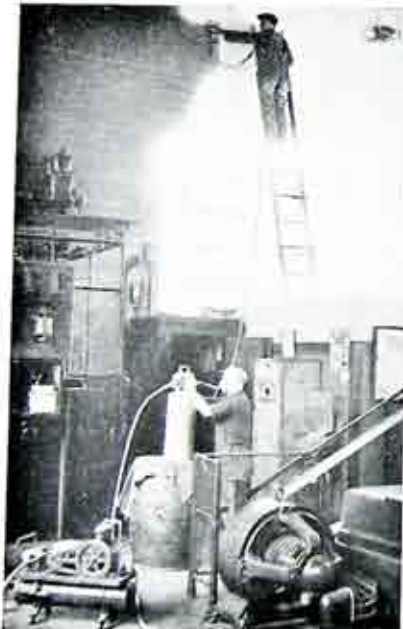
Using the Air Brush at Station 2. Note the Effect of One Coat of Paint thus Applied
