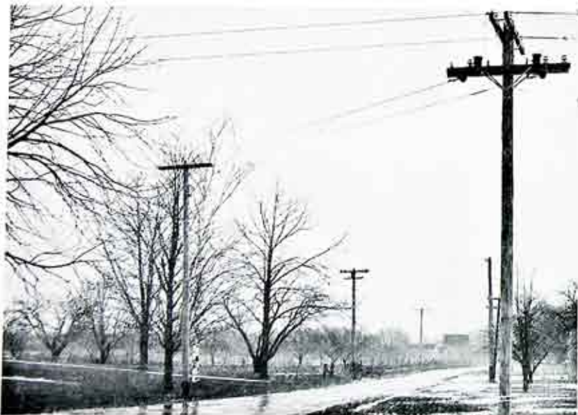
Fig. 4.—Limbs and Branches Close to or Overhanging Wires are a Hazard to Continuous Service.
