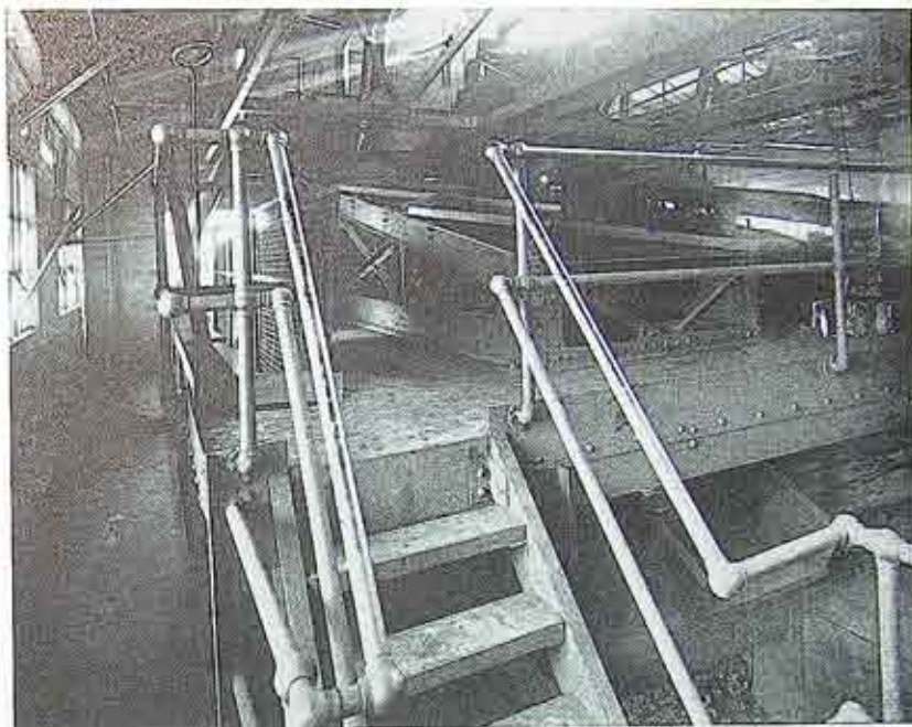
Figure 3. Scene in the Loft of the Coke Bins, Showing Apparatus Used in Sizing the Coke. From this Point the Coke is Chuted to Various Bins from Which it is Emptied into the Trucks Preparatory to Weighing and Delivering to Customers
