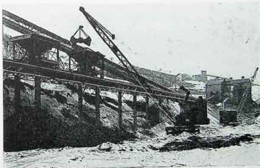
Figure 1. Scene at West Station where two Locomotive Cranes aided by Traveling Hoppers Handle in Normal Periods Approximately 550 Tons of Coke per Day. Interchangeability of Parts in these Cranes Adds to their Efficiency. The Crane in Foreground, recently Purchased, has a Boom 10 Foot Longer than its Mate Shown in the Right Distance
