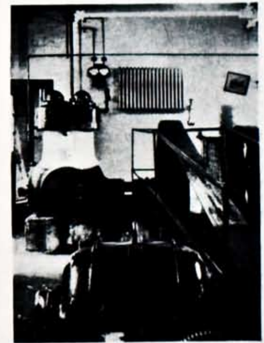
Fig. 3. Electrically Driven Refrigerating Machine at the Big Elm Dairy.
