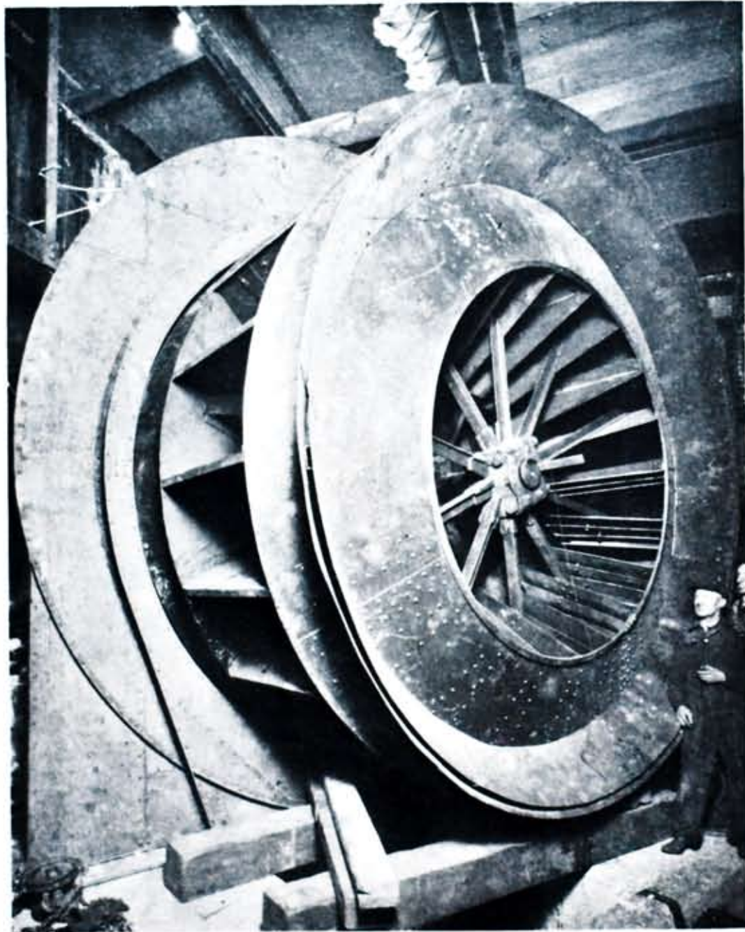
View of the Cinder Fan Wheel Taken Prior to Being Placed in the Fan Casing.
