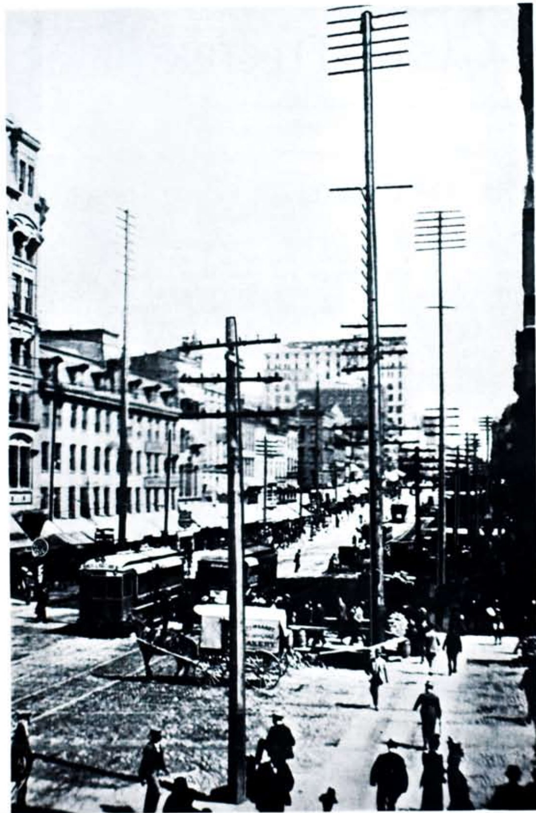
Main Street at Four Corners in 1890, Showing 90 Foot Poles. None of These Poles are to be Seen in Rochester Now.
