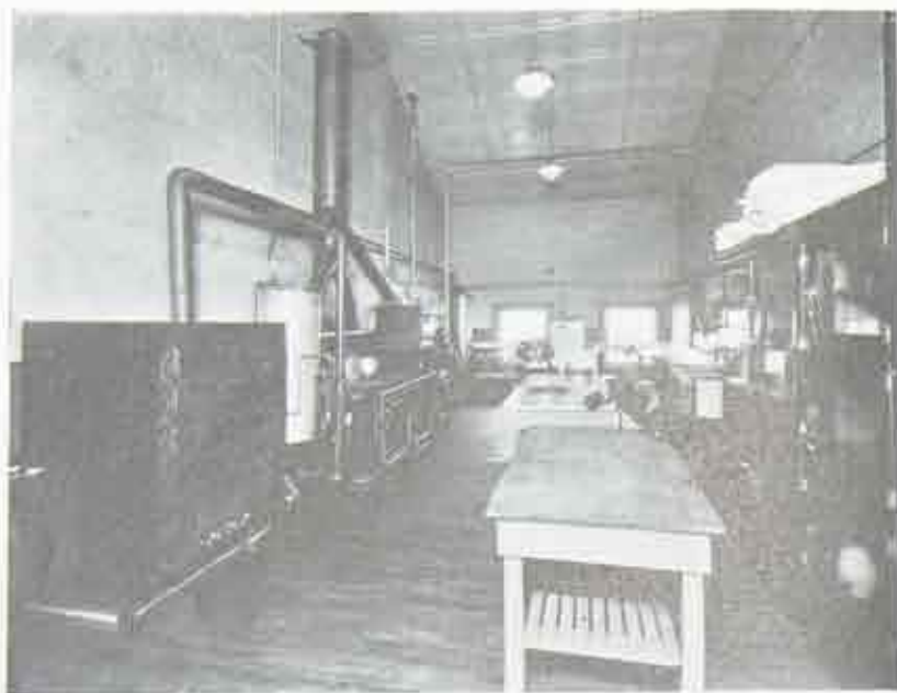
Modern Equipped Kitchen at Andrews Street Commissary.
