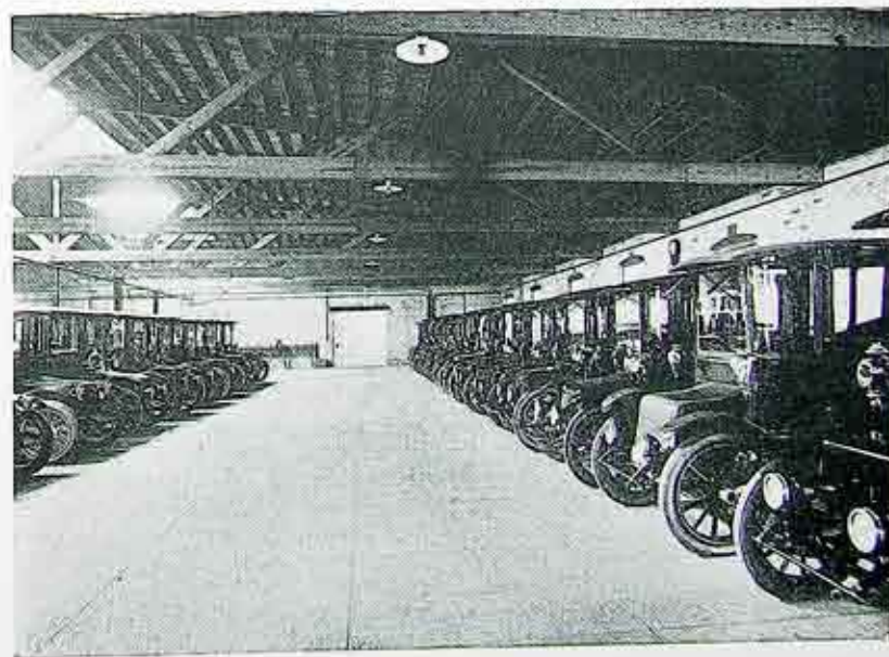
Interior View of Garage.
