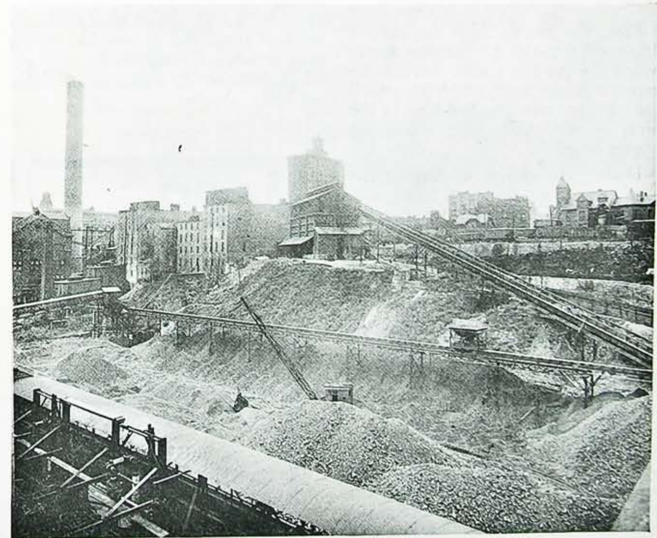
General View of Coke Storage Yard, showing Belt Conveyors and Crane with Storage Building in Background.
