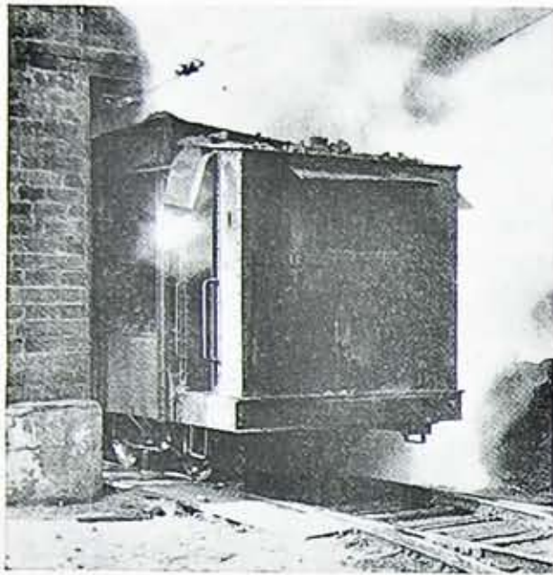
Coke Car leaving Building.
