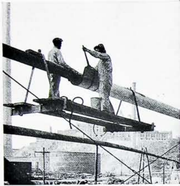
Fig. 3. Working on Scaffold.
