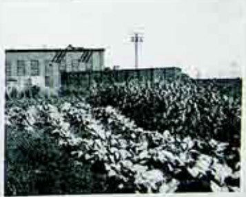
THE CONCRETE POLE YARD ALSO SERVED AS A GARDEN SPOT.
