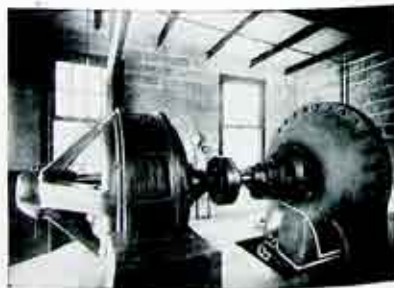
Fig. 7. Sixteen inch single stage centrifugal pump direct connected to 200 horsepower electric motor installed in building shown in figure 6.
