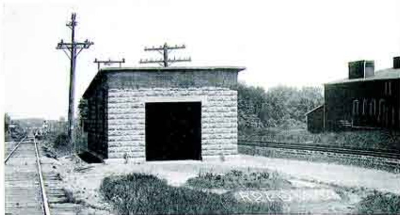
Fig. 6. Rochester and Lake Ontario Water Company's "booster" plant installed near the Ridge Road on the right of way of the Buffalo, Rochester & Pittsburgh Railway.
