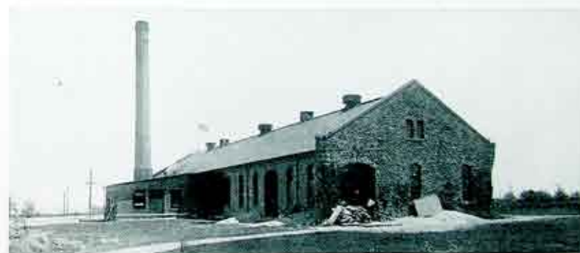
Fig. 1. View of Rochester and Lake Ontario Water Company's Pumping Plant located on the shore of Lake Ontario about one and one-quarter miles west of Lake Avenue, Charlotte. The reader is looking east toward the Lake. Projection is addition recently built on.
