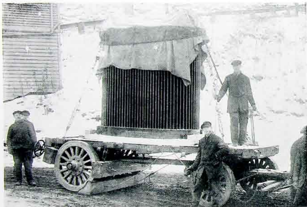
Picture of eleven ton transformer after it had been transported down the Falls Street Hill.
