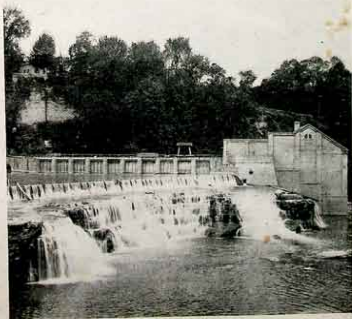
Station 15 and Old Dam at Middle Falls
