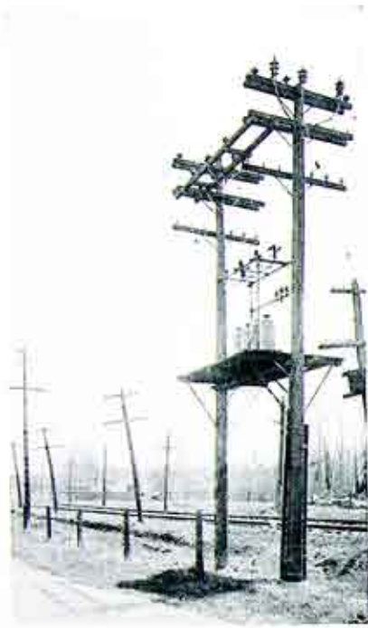
Fig. 2. 11,000-volt line rising from underground at Rockwood Street. From this point it is carried overhead to East Rochester
