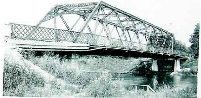
Four inch pipe crossing canal bridge on Church Street, Fairport. This pipe is black steel with welded joints and is fastened to girders under the sidewalk.
