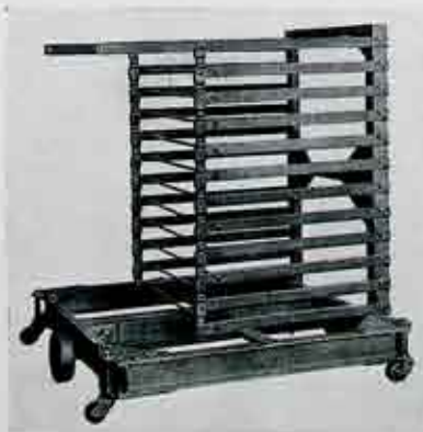
Fig. 3. Truck (capacity 12 plates) used for hauling piano plates into the ovens
