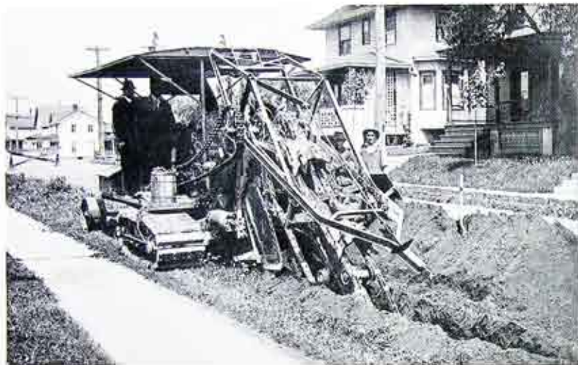
Fig. 4. Trenching machine which was used for digging the trenches
