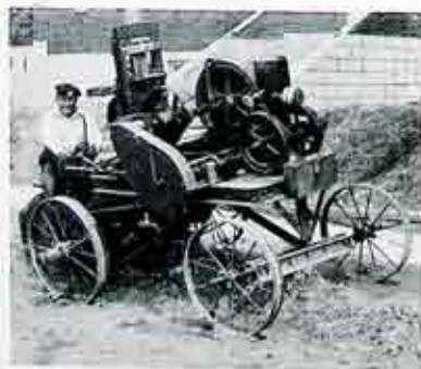
Fig. 5. Tamping machine at work
