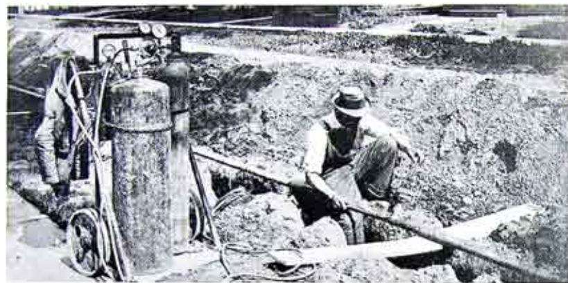
Fig. 2. Welding pipe prior to dropping it into trench at East Rochester
