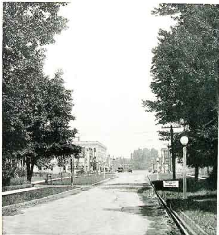
Main Street, East Rochester, near Commercial Street
