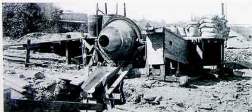
Two-thirds-yard concrete mixer belted to 10 H.P. motor under platform. This is an ideal drive, especially where safety and efficiency are important factors.
