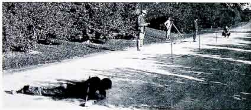
Precise measurement of "base line": Note standards used to keep tape level. Spring balance used so that pull on tape will always be the same as under original U. S. test. Thermometer attached to tape so temperature correction can be made.
