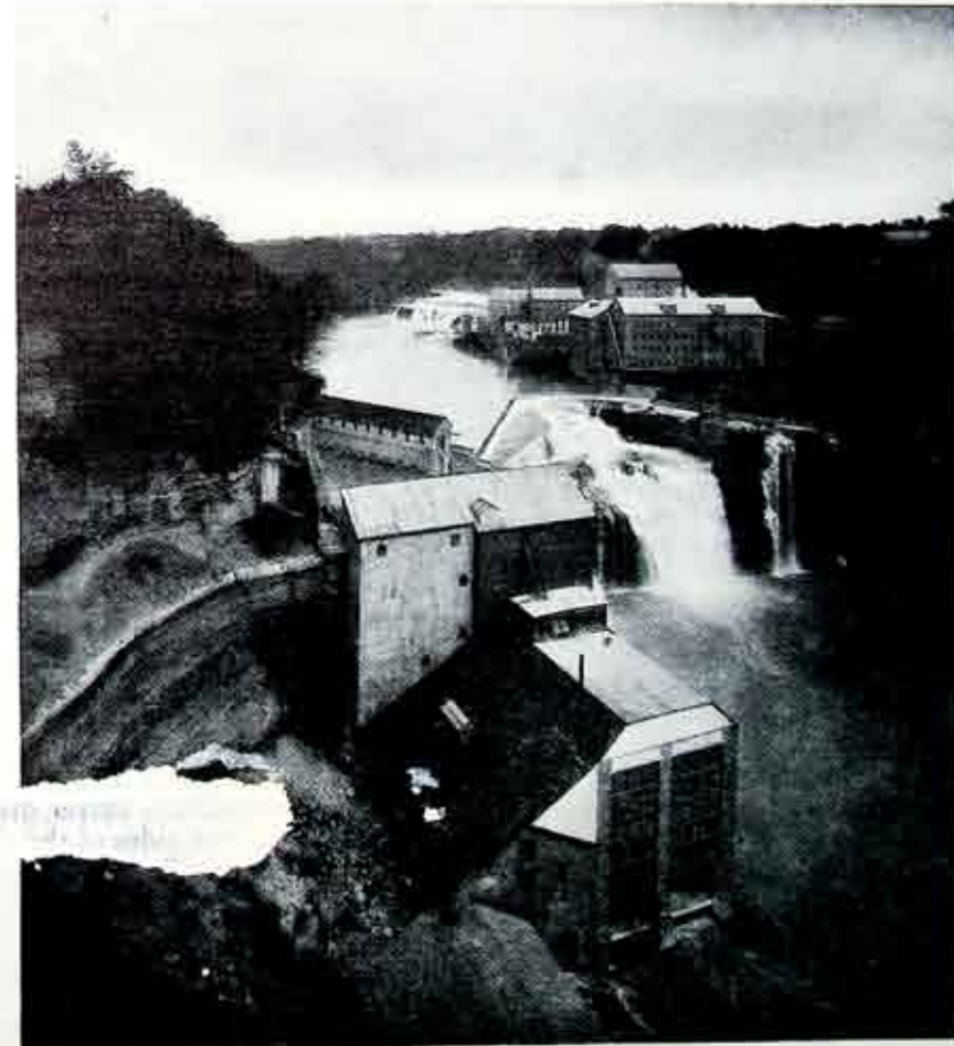
Station 5 at Lower Falls Where New Station Will be Built
