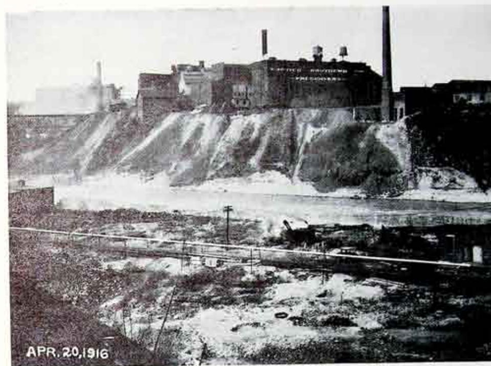
Preparing Site for New Gas Works,—Station "B"
