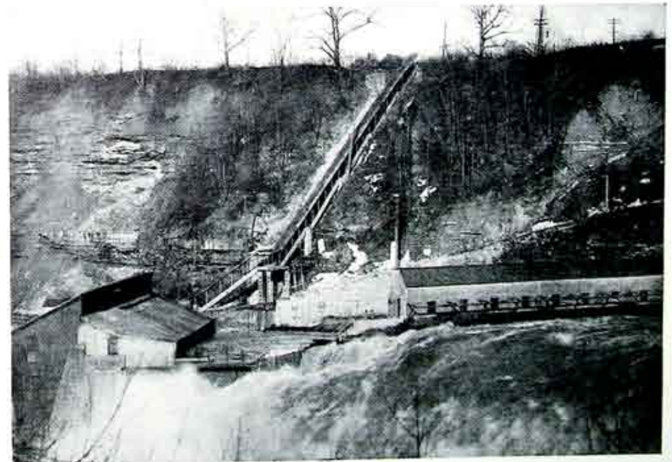
Flood at Gate House of Station 5
