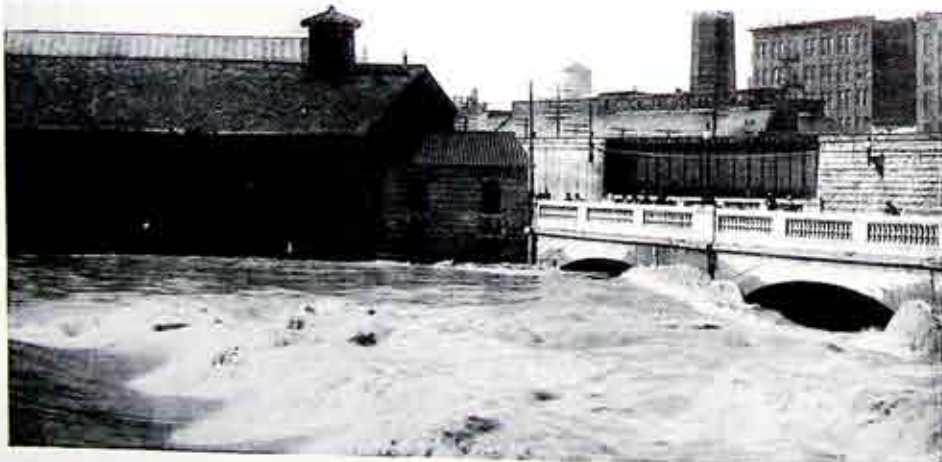
Upper—Genesee River at Elmwood Ave. Bridge, near Station 33. Middle—River above arches of Erie Canal Aqueduct near Station 6. Lower—High water at Front Street Garage and Central Ave. Bridge
