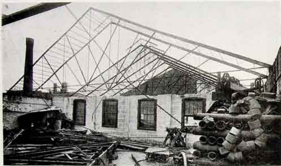
Fig. 1. View of Old Roof Trusses
