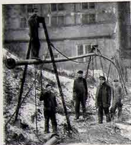
Erection of Steam Main
