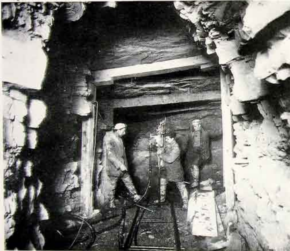
Section of Tunnel near Plymouth Avenue
