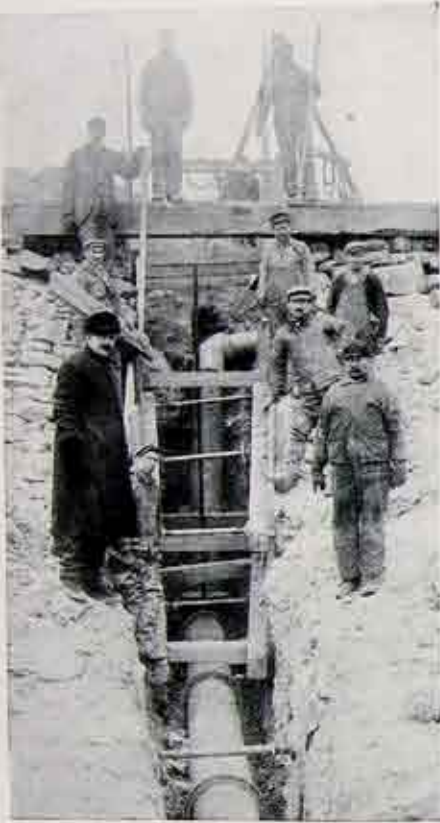
Special Construction Near Culver Road.
