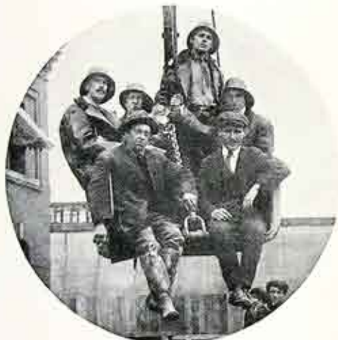
Ready to be Lowered
