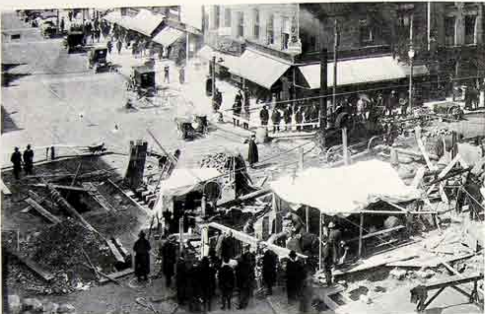
Electrically Driven Pumps Used to Pump Out Main Street Cave-in.
