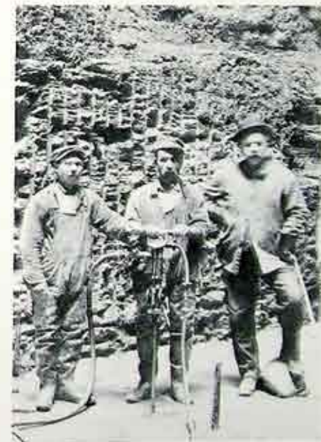
Small Drill Used in Excavation of Pit for New 10,000 KW Steam Turbine.
