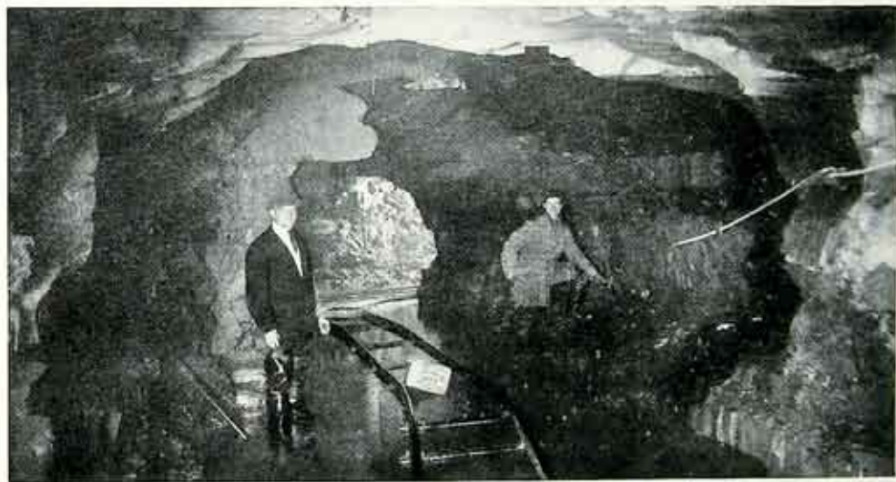
Intersection of Tunnel at Main and Front Streets
