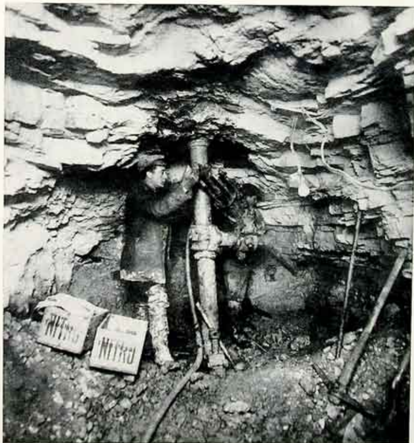
Tunnel Heading—Main and Front Street Sewer
