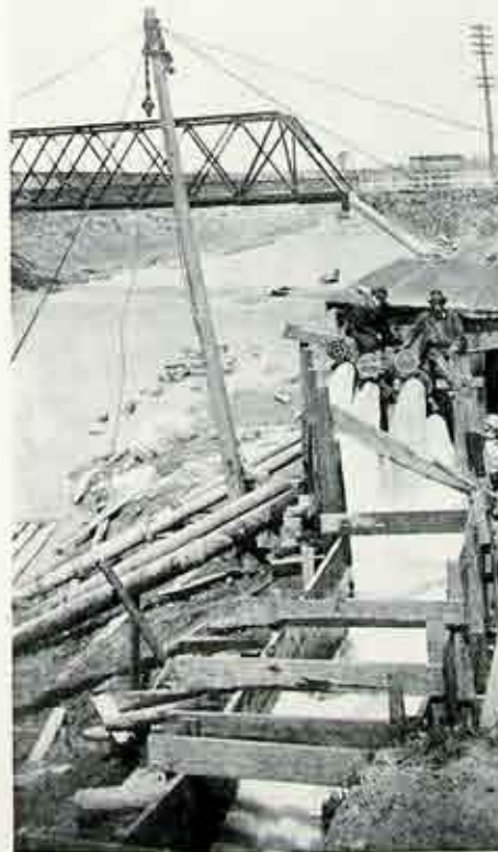
Fig. 1. Four electrically-driven 10-inch pumps discharging into flume.
