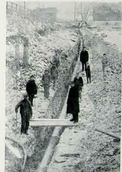
16 inch Gas Main Under Bed of Canal at Widewaters
