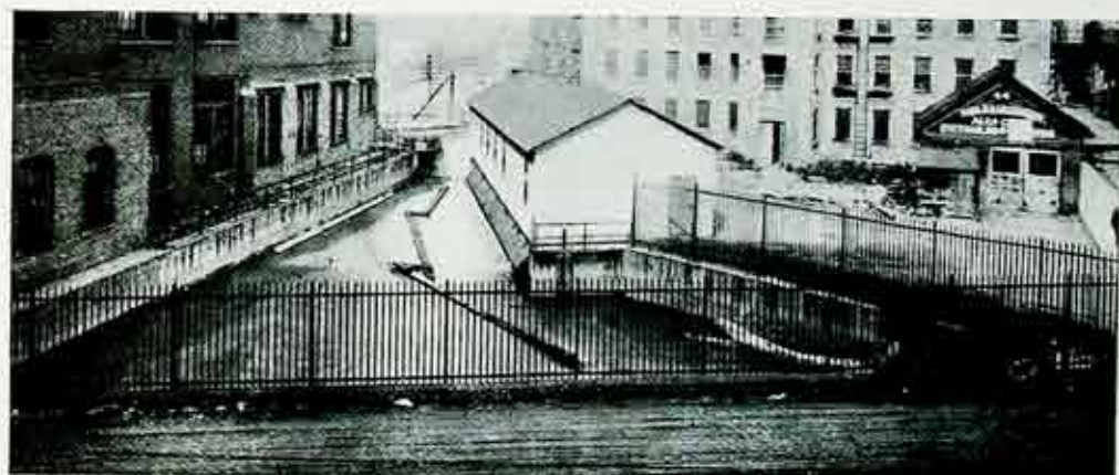
Forebay and Gatehouse of Station 2-A
