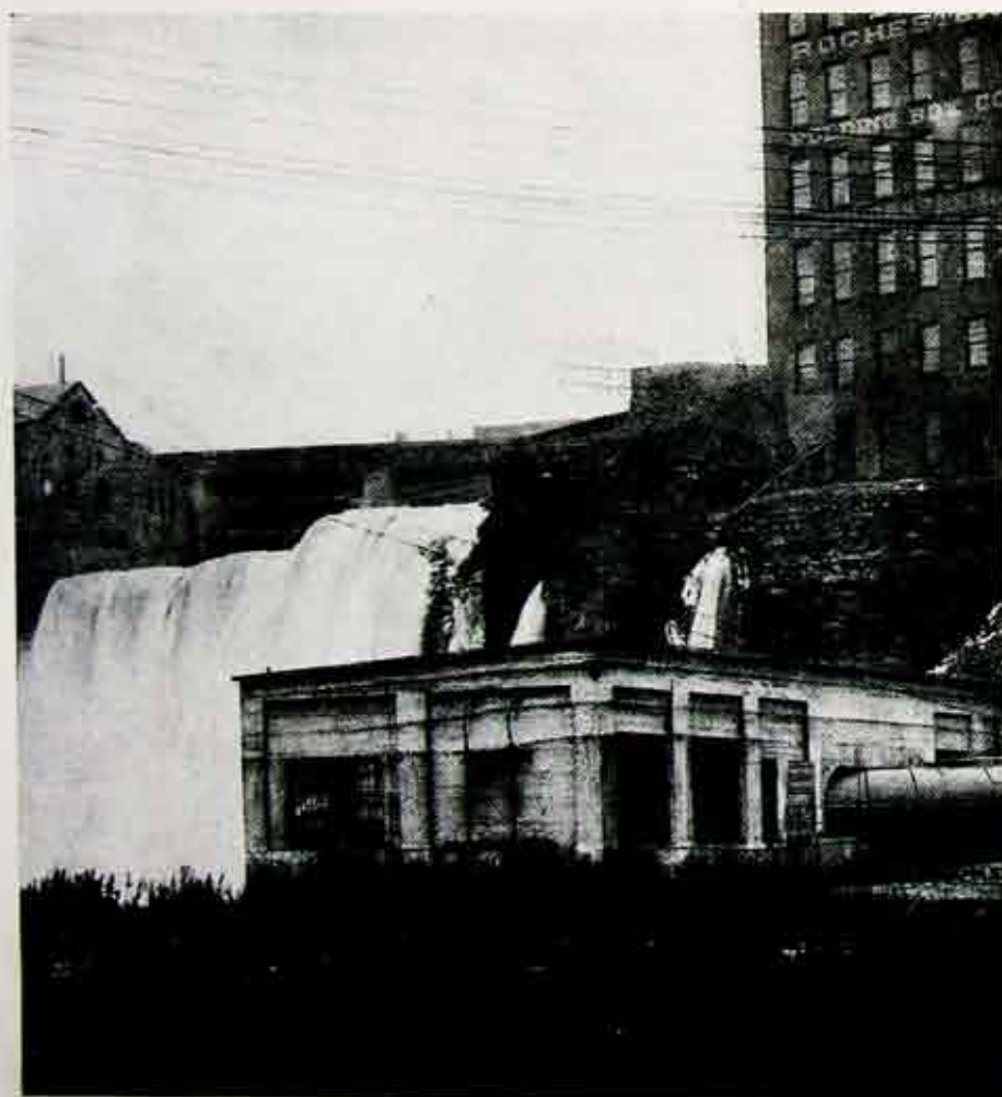
Station 2-A at Upper Falls
