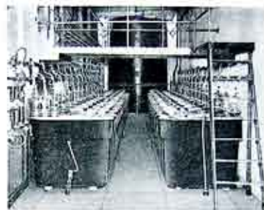
Fig. 3. Equipment of Oxygen Generators in Operation
