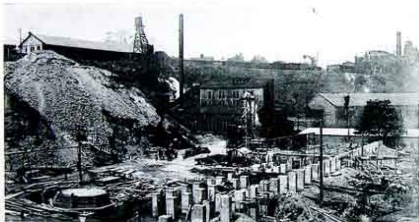
Station B. Site. Hill at left to be washed onto the low ground toward River at right of picture.
