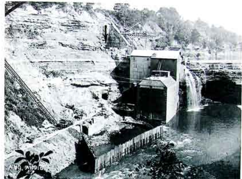
Fig. 2. Station 5 showing outlet of tunnel. Arrow shows location of surge tank. Coffier dam built to permit work on new building and tail race.
