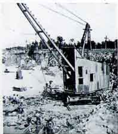
Shovel and Hoist
