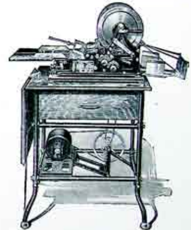
Motor-driven Mimeograph—Prints copies through Dermatype stencils made on typewriter.
