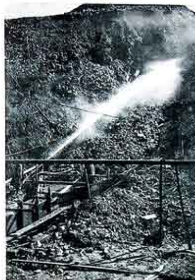
Fig. 2. Hydraulic Sluicing at Station B; water under 150 pounds pressure
