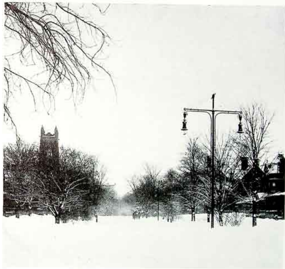
Portsmouth Terrace after Construction of Subway
