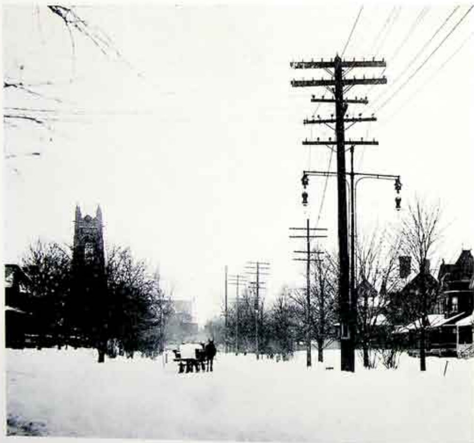
Former Overhead Line Construction on Portsmouth Terrace
