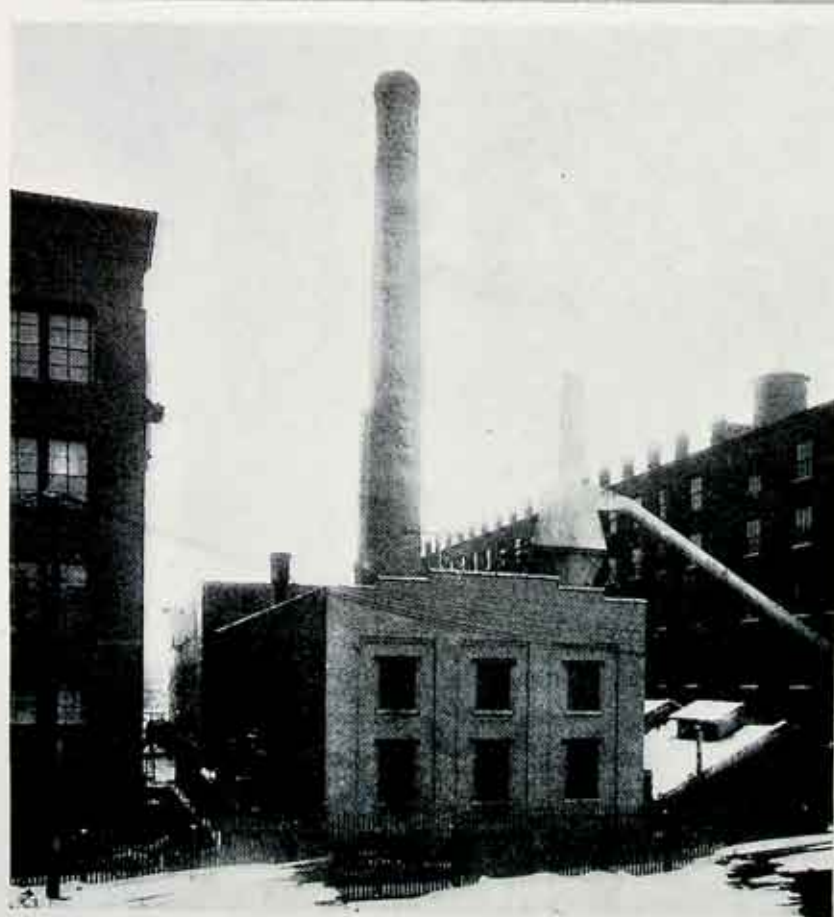
Station No. 35 on Litchfield St.
