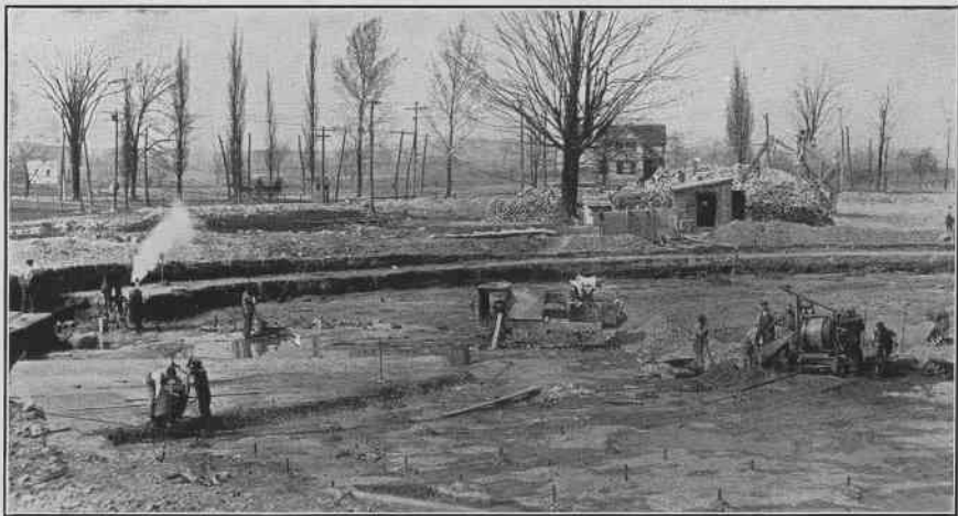
Figure 3. Average Depth of Excavation 4 Feet. Below This There Is a Solid Rock Foundation, Levelled on Top with a Concrete Pancake.
