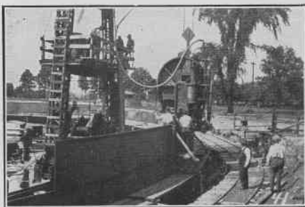
Figure 7. 150 Ton Hydro-Pneumatic Riveter at Work.
