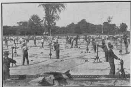
Figure 6. Lowering Bottom of Tank, June 14, 1913. 162 Men Required for This Job.
