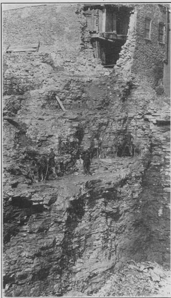
Figure 1—Using Electric Drill on a Narrow Ledge.
