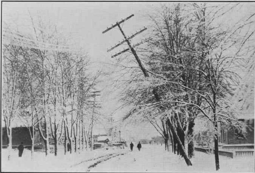
The heavy ice-laden branches of the trees in Murray Street bore down this pole. The wires on the lower cross-arms are responsible for its condition. Many poles were found like the one shown above, demonstrating the desirability of getting poles and wires off the streets, especially where there are shade trees.
