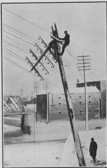
One of five poles near Canal Weighlock on South Avenue which collapsed during the storm. This pole was doubled guyed, and the point of breakage occurred between the points of guy attachment, evidence of the tremendous crushing strain imposed by the ice and snow load. This line of poles is known as the Canal line, and carries two 3-phase power circuits and twelve arc circuits out of Station No. 6 to the east part of the city. A force of linemen under J. Cox and J. Downs had five new 60-foot poles in place and all circuits running day after storm.
