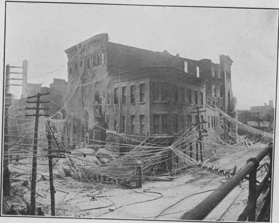
Fig. 3. Corner Central Avenue and North Water Street, showing condition of poles and wires after a fire in 1902.
