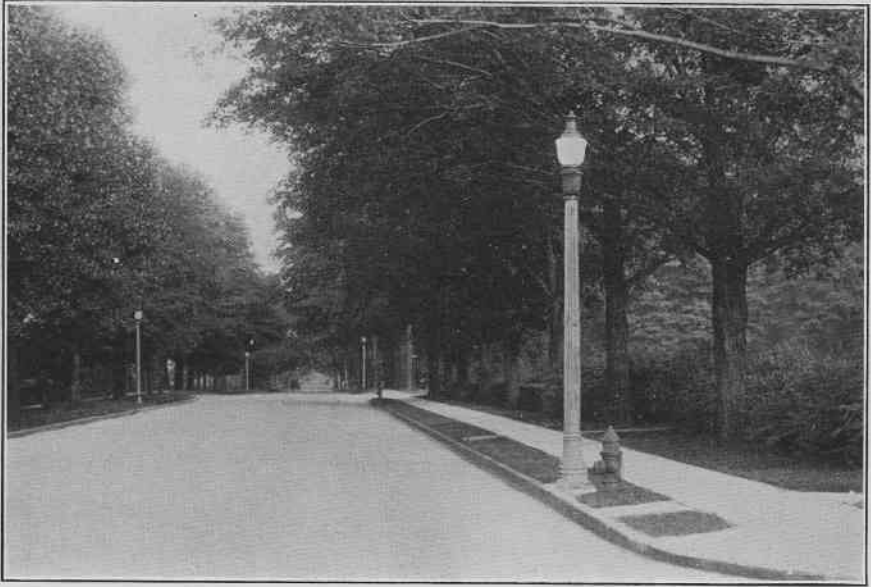
Daylight picture, showing arrangement of new East Avenue lamp posts. The lamps are "staggered" 200 feet apart. Each lamp is provided with a switch or cut-out to enable repairs to be made in safety. The switch is located in base of lamp, access being had through a door placed therein.
