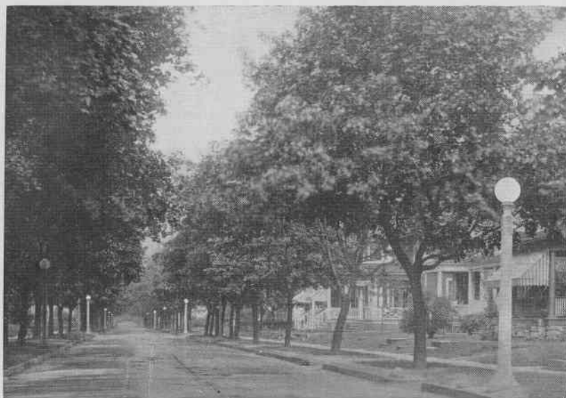
Fig. 2. Concrete Tungsten Standards and Cast-Iron Luminous-Arc Posts on Warwick Avenue.
