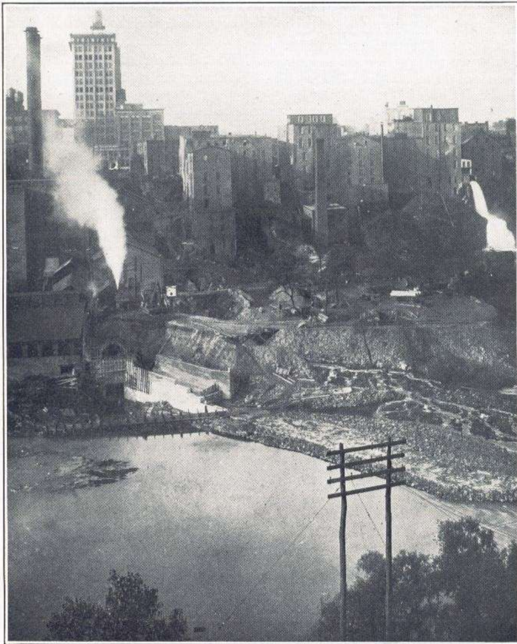
General view of yard back of No. 3 Station, showing new intake on River below old Platt Street sewer. New sixteen story Eastman Building in background.
