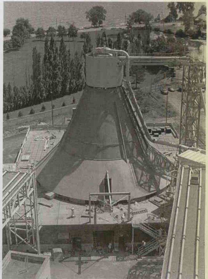
>> The conical-shaped splitter building as part of the refuse-derived fuel burning project during the 1970s and 1980s.
